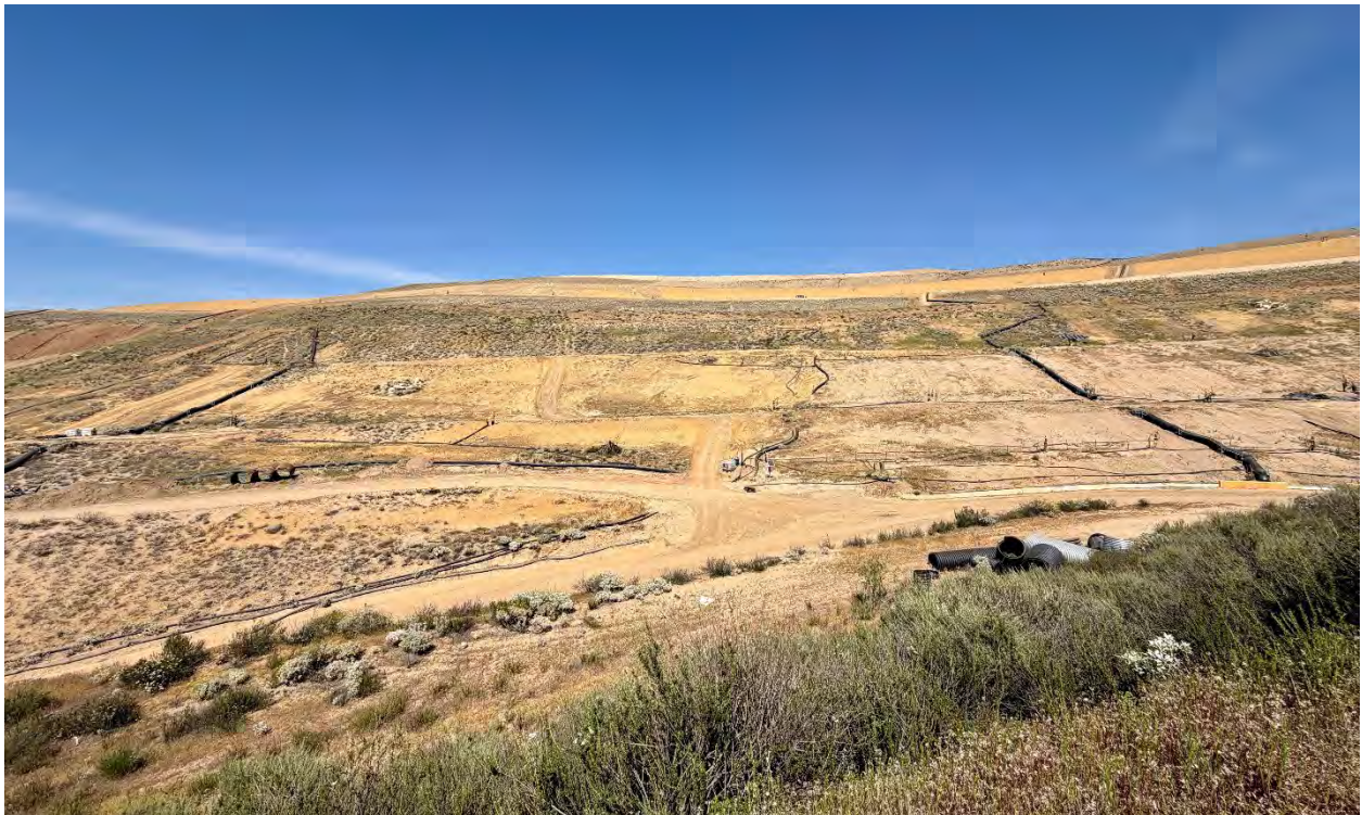
Photograph 8. The center part of the landfill is an active construction zone, March 22, 2026.
