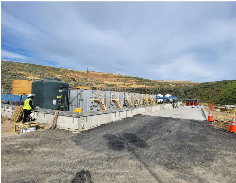
Photo 1: The black polyethylene tank is the proposed backwash storage tank, and the seven gray frac tanks are the proposed hazardous frac tanks.
