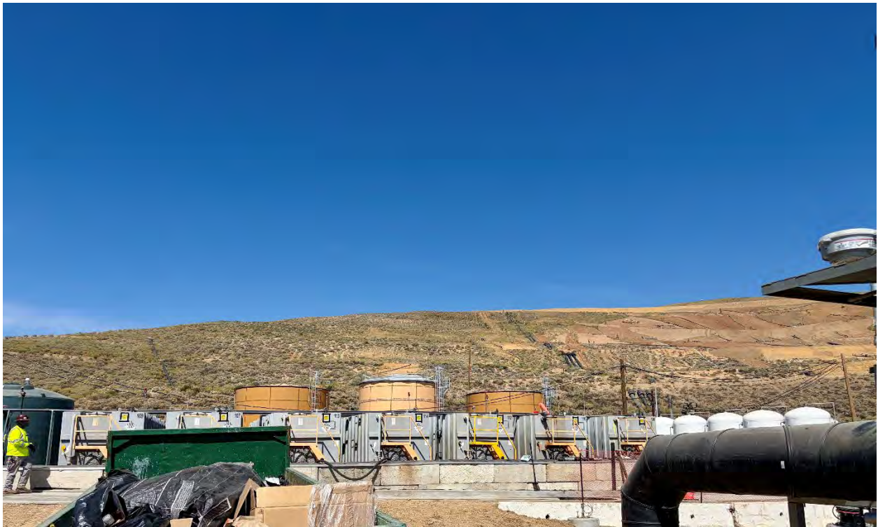
Photograph 4. The west end of the landfill, March 22, 2026.
