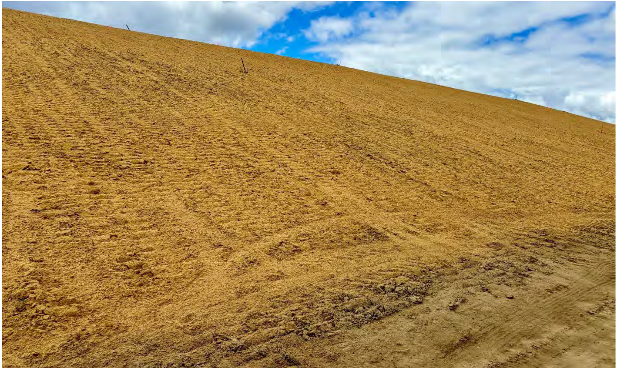
Photograph 16. A seeded slope in Phase D2, May 5, 2026.
