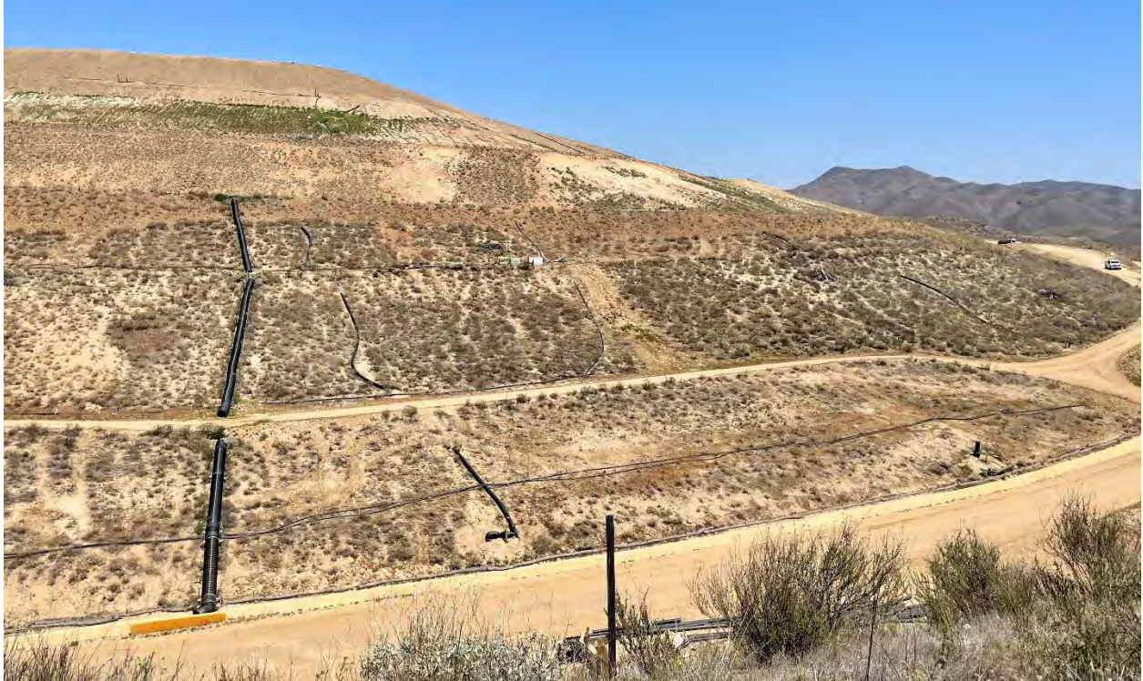
Photograph 11. The east end of the landfill, April 28, 2025.
