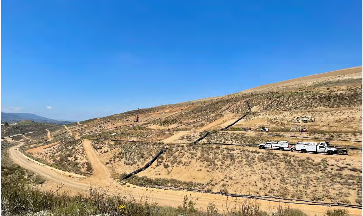
Photograph 5. View of the western slopes, April 28, 2025.
