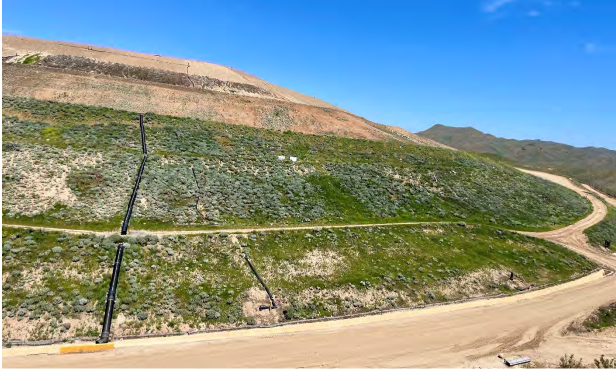
Photograph 11. The east end of the landfill, April 15, 2024.
