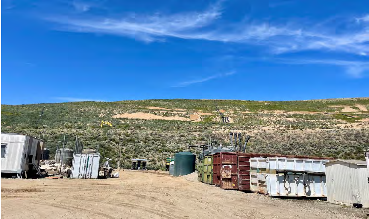
Photograph 3. The west end of the landfill, April 15, 2024.
