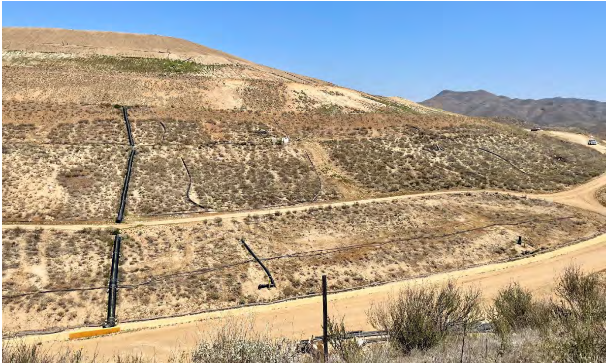
Photograph 12. The east end of the landfill, April 28, 2025.
