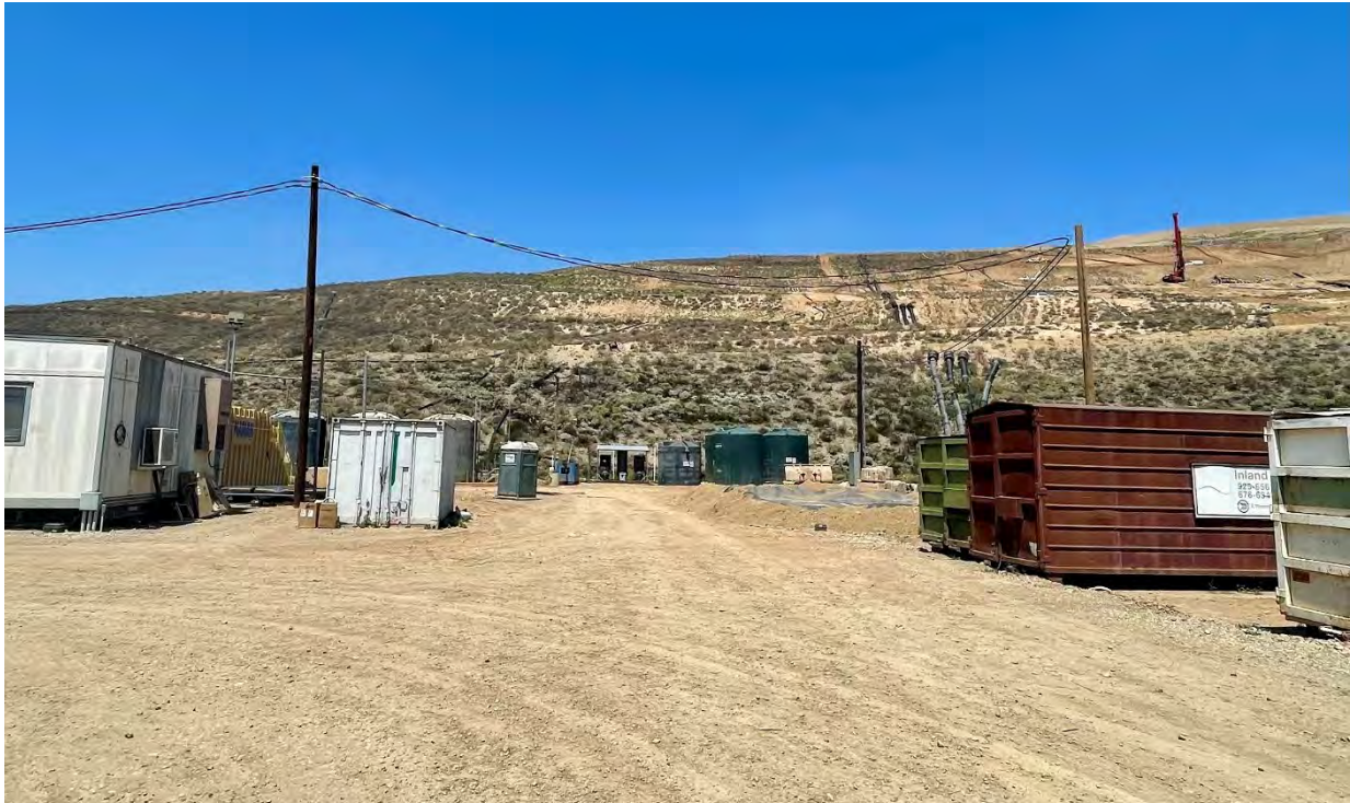
Photograph 4. The west end of the landfill, April 28, 2025.
