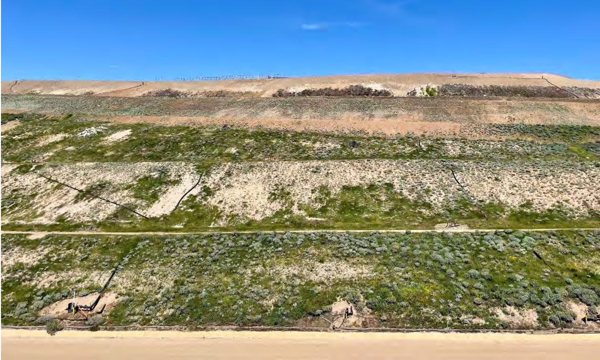
Photograph 9. Phase C1 rock outcrop and Y-shaped pipes, April 15, 2024.
