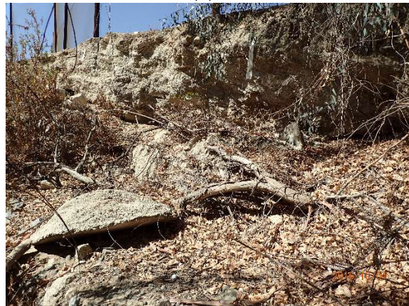
Photo 34. The left bank near the Temescal Wash confluence. Note the vertical exposed bank and concrete blocks on the slope. Reach 1. 10/4/16.
