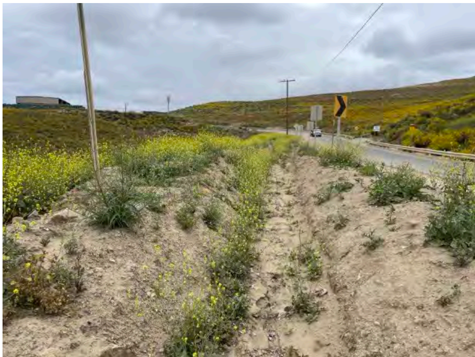
Photo 34. Roadside ditch (D-16) that conveys storm water runoff from the North Old Maintenance Shop site to an offsite detention basin, looking northeast. (May 10, 2023)
