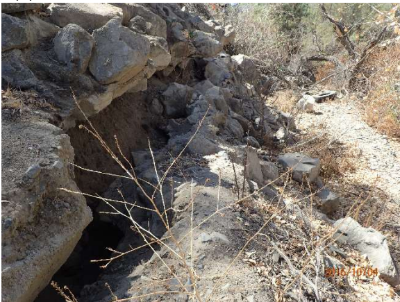
Photo 33. View upstream of the right bank near Temescal Wash confluence. Note the failure of the grouted rip-rap. Reach 1. 10/4/16.
