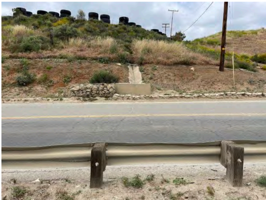
Photo 18. Brow ditch (D-4) that drains into small detention area with no outlet, looking west. (May 10, 2023)
