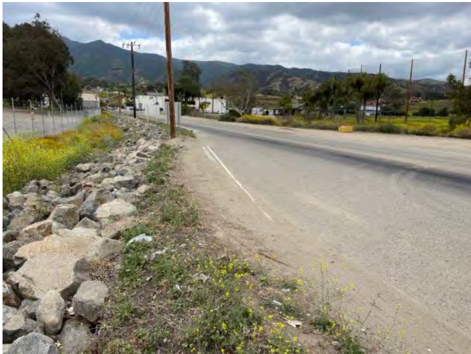
Photo 12. Roadside ditch (RD-1) lined with riprap along Dawson Canyon Road, looking southwest. (May 10, 2023)
