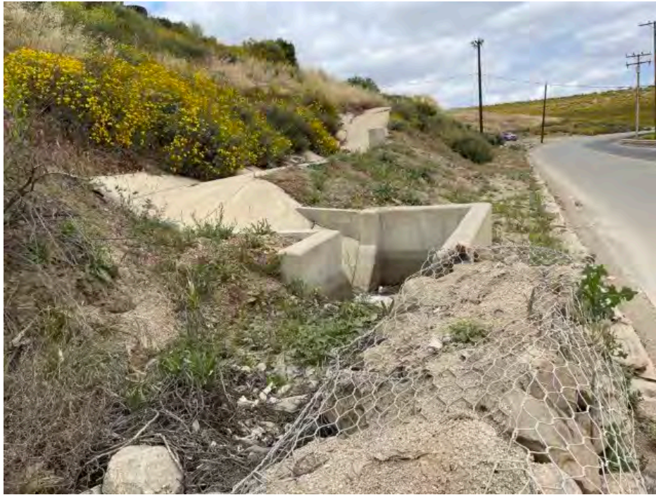
Photo 17. Brow ditch (D-3) that drains into small detention area with no outlet, looking northwest. (May 10, 2023)
