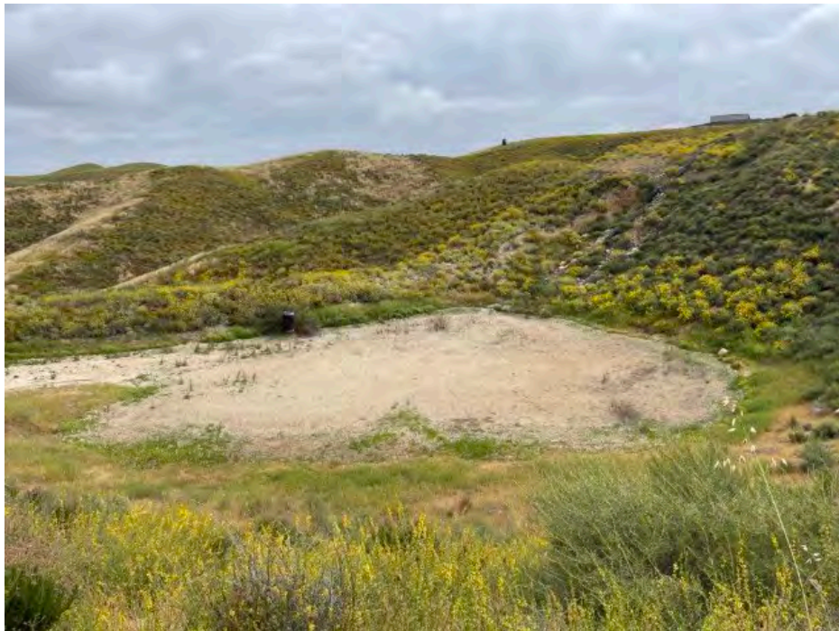
Photo 36. Offsite detention basin southwest of the North Old Maintenance shop that receives water from pipe that drains a roadside ditch (D-16), looking northeast. (May 10, 2023)
