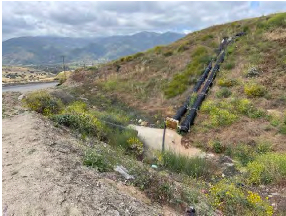
Photo 21. Offsite pipe that drains into small detention area with no outlet, looking southwest. (May 10, 2023)
