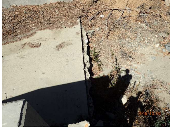
Photo 32. Box culvert downstream apron. Note the scour on the downstream face. Reach 1. 10/4/16.
