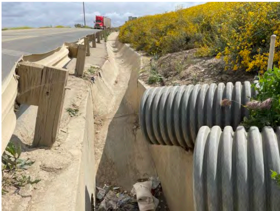
Photo 30. Pipes on adjacent slope draining into roadside ditch (D-13) along Dawson Canyon Road, looking northeast. (May 10, 2023)
