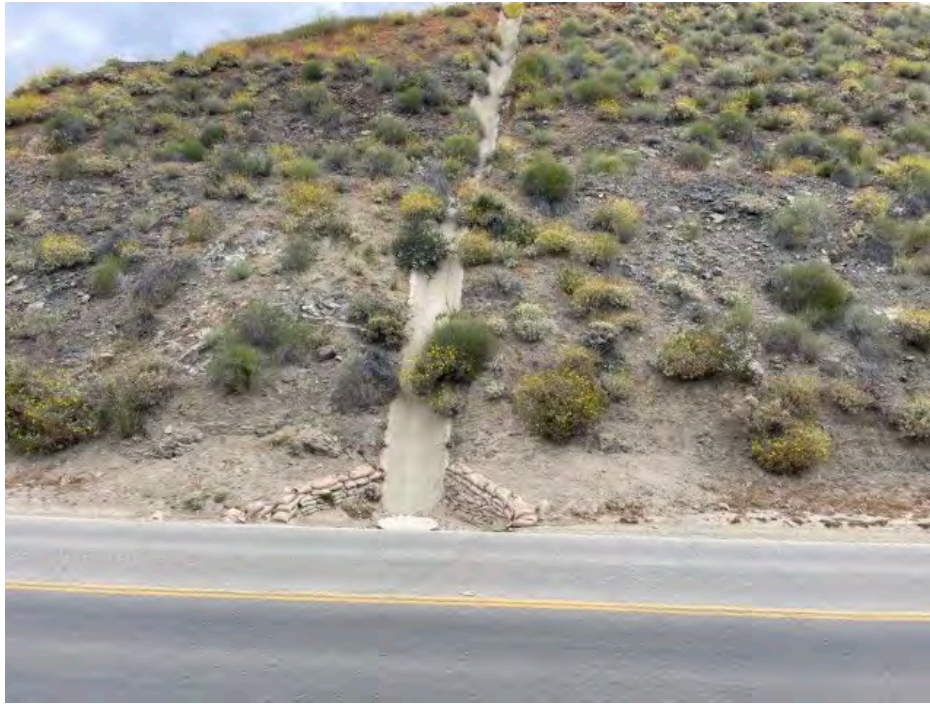
Photo 13. Brow ditch (D-1) on slope that drains into pipe/culvert inlet, looking northeast. (May 10, 2023)
