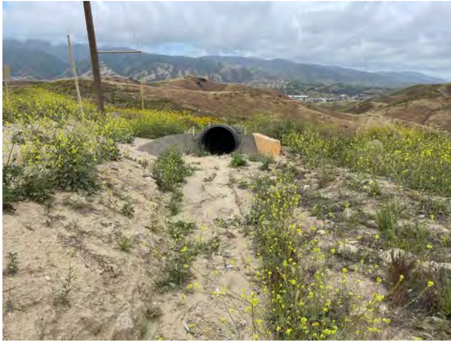
Photo 35. Pipe inlet that drains roadside ditch (D-16) to an offsite detention basin, looking west. (May 10, 2023)
